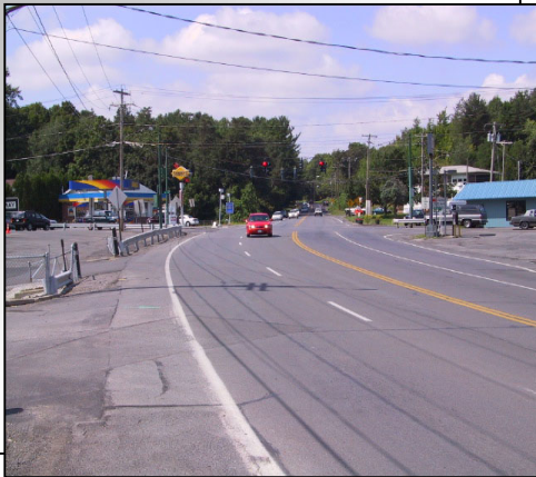
This 5-leg intersection was reconfigured with turn lanes for all approaches. Curbed islands eliminated the "free for all" access to parking lots.
