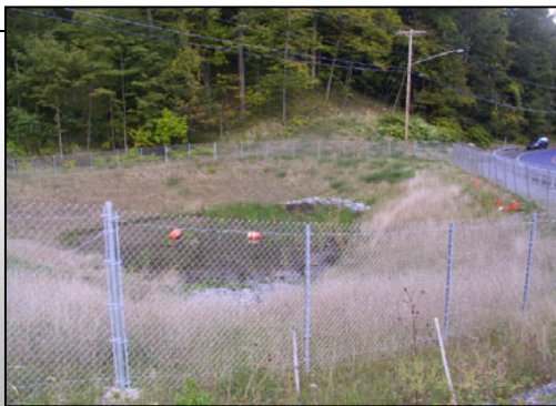
This detention basin provided a solution to the increased runoff from the NYS Route 173 project at the west end.
