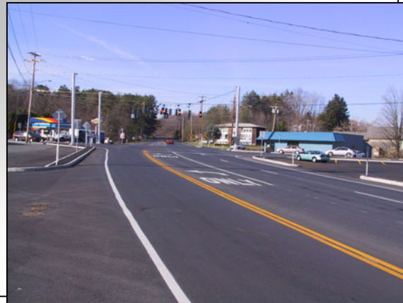
This 5-leg intersection was reconfigured with turn lanes for all approaches. Curbed islands eliminated the "free for all" access to parking lots.
